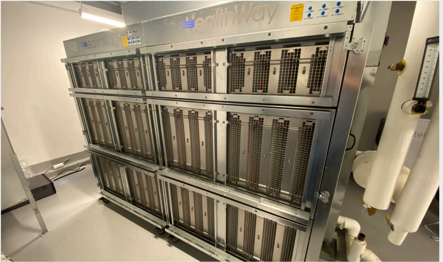
After: HealthWay 2000/1000IL Modular Array Retrofit | Installed Array
