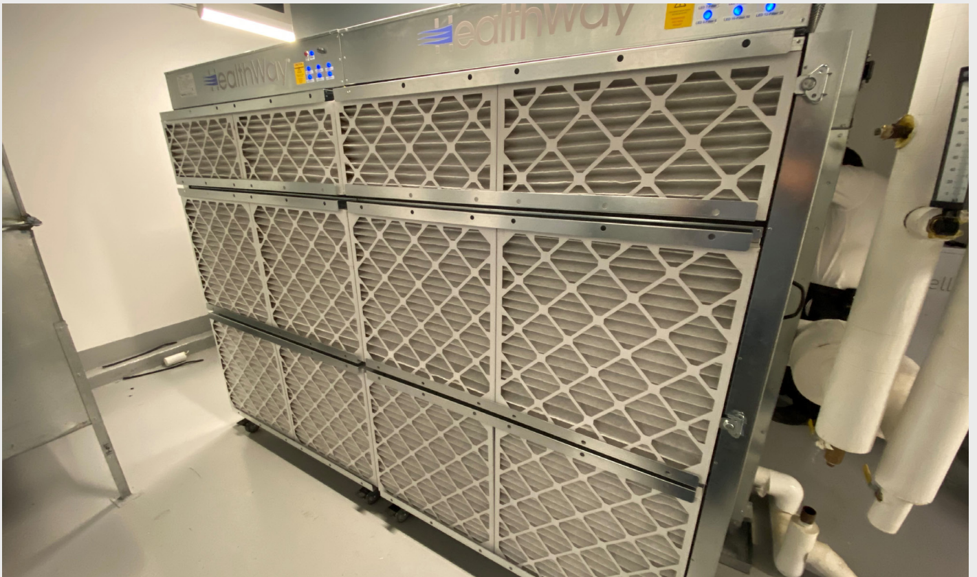
After: HealthWay 2000/1000IL Modular Array Retrofit | Filter Lights and Pre-Filters
