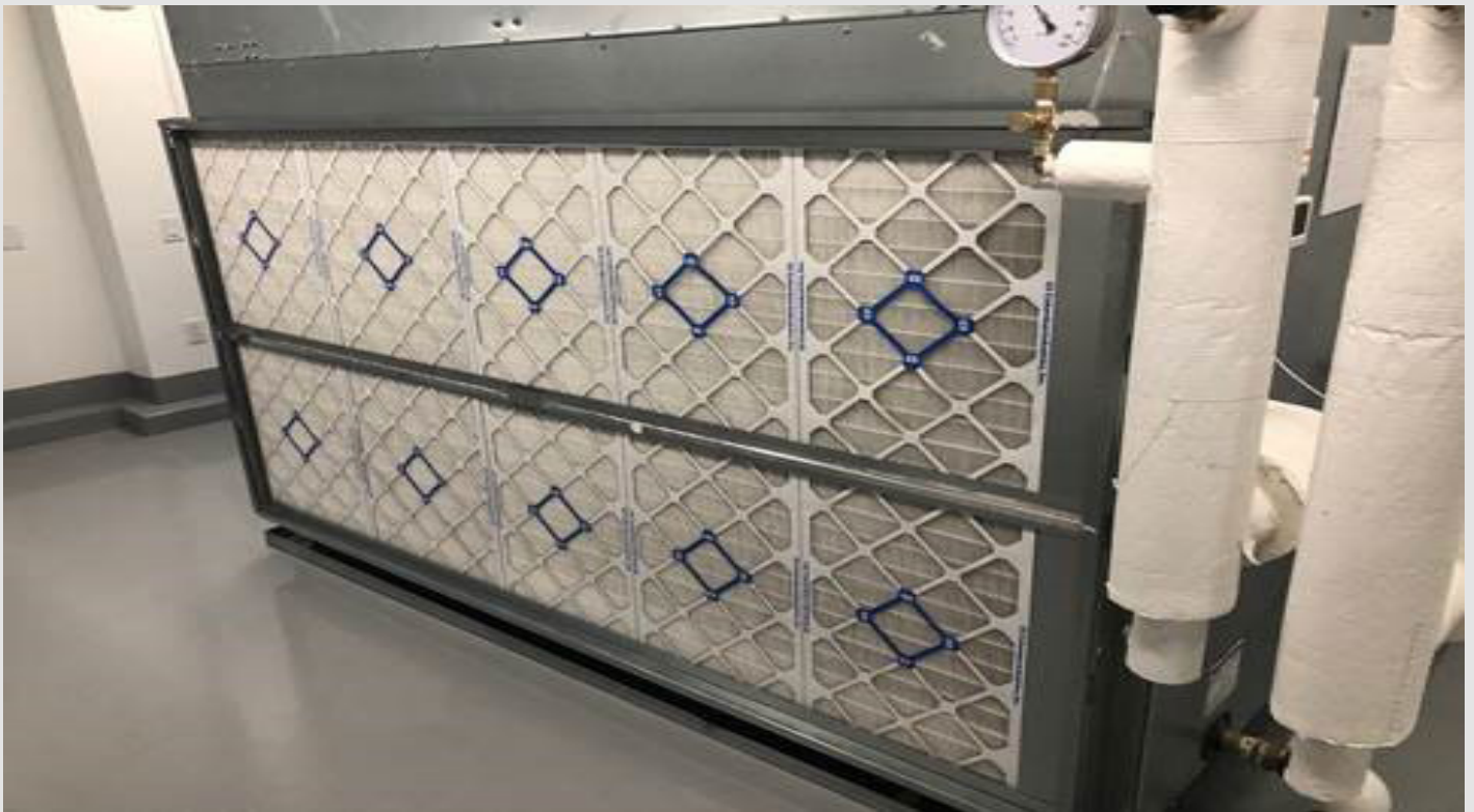
Before: Pre-existing AHU with MERV 15 Filters
